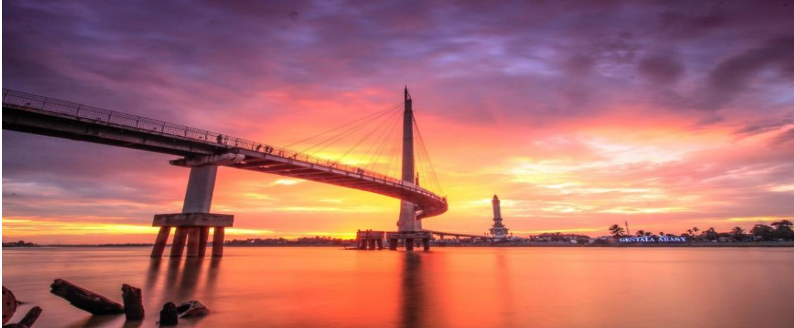
Figure 4. Gentala Arasy Bridge
